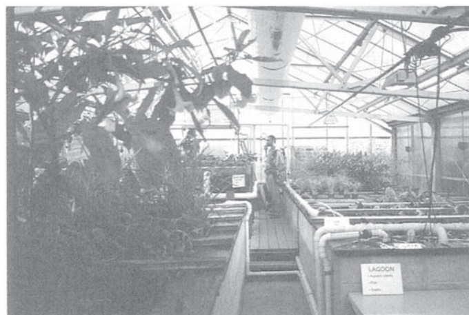
Fig. 4. Solar aquatic “Living Machine.” Hydroponic gardening (for horticulture) part of nutrient waste recovery system utilizing sewerage waste from an office building, also cleaning water for landscaping. John Todd, Designer.
